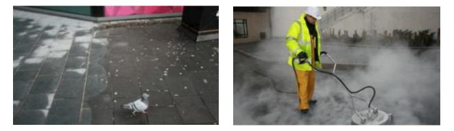
The DOFF is a high-pressured steam cleaning system whereby you can control the temperature of the steam to tackle 'hard to clean' surfaces. Because it uses steam, it's also environmentally friendly.
