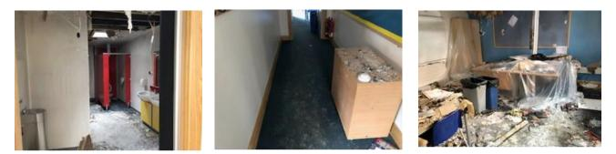
The walls (constructed by stud partition and plaster in most rooms, while others are blockwork and plaster) were wet and required drying. The floor slabs were also wet as these areas had been subjected to abnormal amounts of water ingression. The ground floor construction consists of carpet tiles, floor screed, a concrete base, insulation, DPM (damp proof membrane), and hardcore. Some areas also had moisture barriers.
